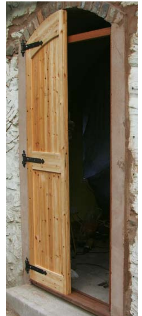
▲ Pic.4 Phil used DIY store strap hinges onto mortared frames to fit the shutters
